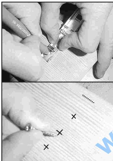
EN Whilst ensuring it remains in this position (2 - 3 mm below the mark) mark off the holes for the 3 screws inside the fastening piece E2.
