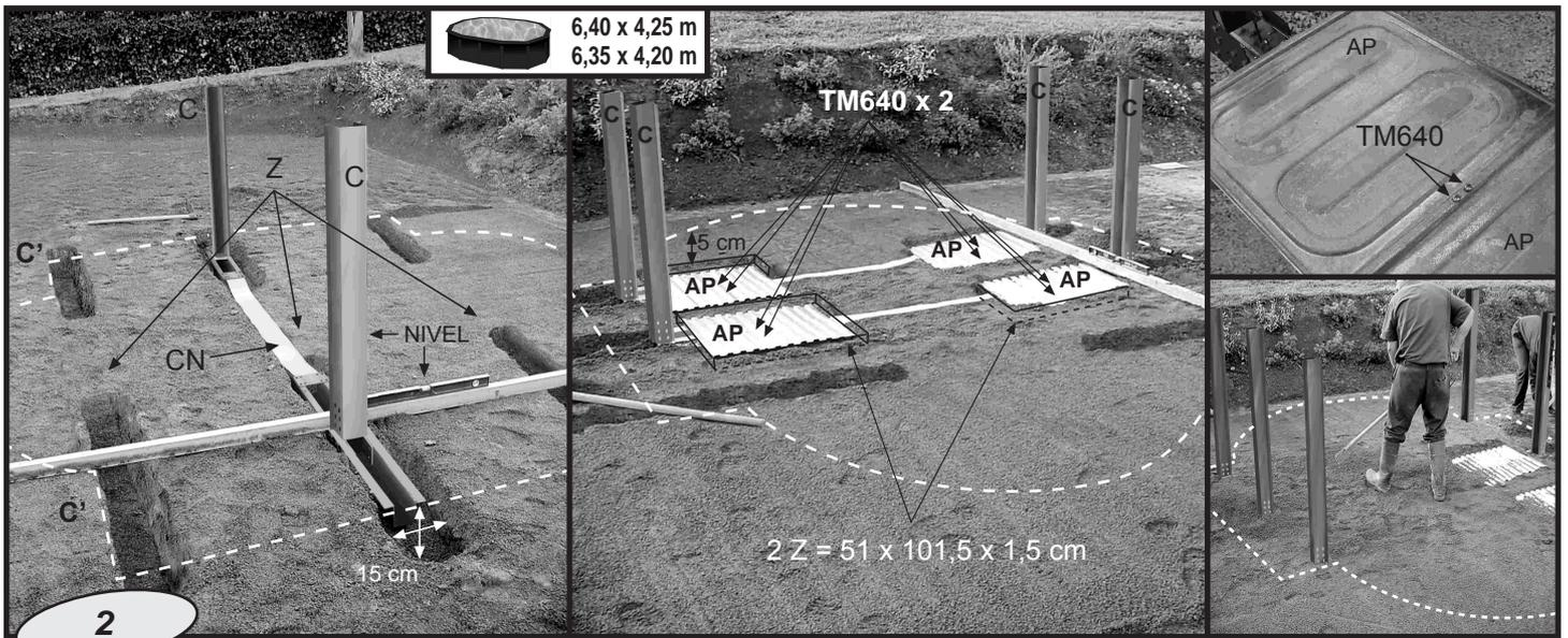
**EN** **VERY IMPORTANT:** When the assembled structures (each consisting of 2 uprights with a strut, the number depending on the type of pool) are inserted, they must be wedged up so that the uprights are at the same level, before and after the trenches are filled in. It is advisable to place a slab or tile beneath each upright to help it withstand the weight of water when the pool is filled.
