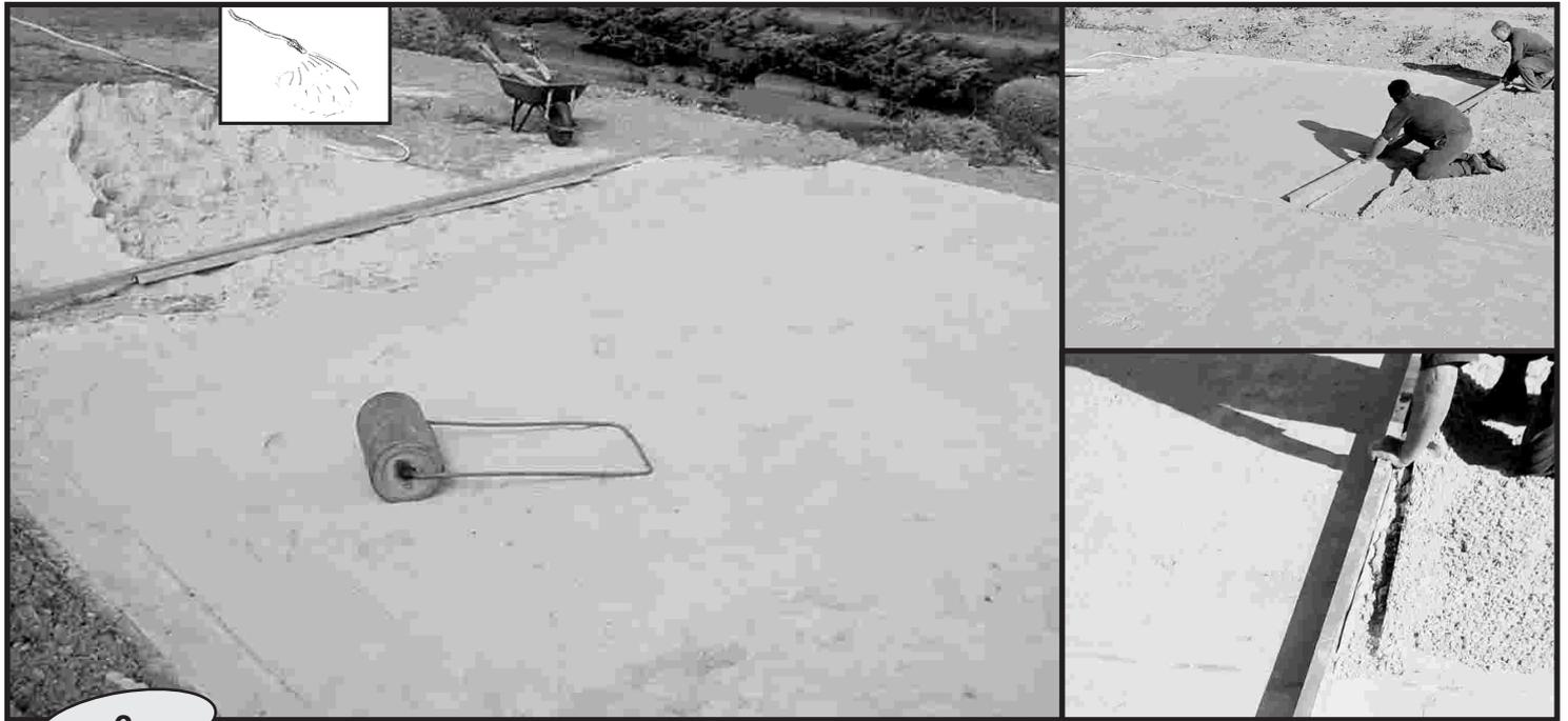
**EN** **Finishing:** On the cleaned and levelled ground, spread a light coat of sieved sand (max. 1cm). Water and compact it (with a garden roller). Check that it is well levelled. Do not use the sand to level the ground. The finishing has to be perfect.
